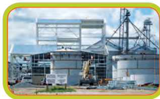
Construction of the Warden Crusher
