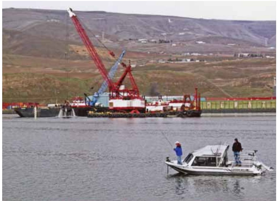
Port of Lewiston Dredging
