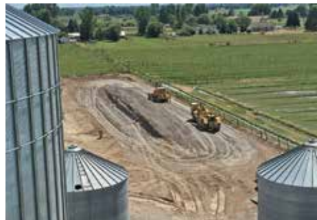
Improvements at the Moreland location
