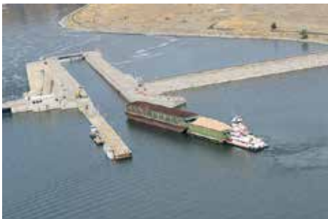
Aerial view of Lower Granite Dam and navigation lock
