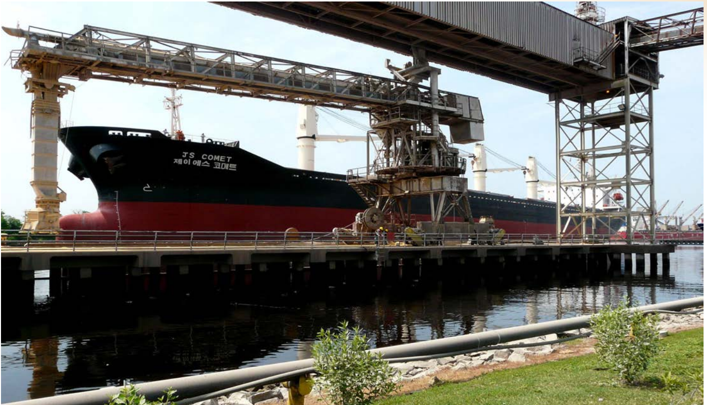
Perdue Export Elevator, Norfolk, VA. Bulk freight rates are expected to "normalize" with freight rates back at least at moderately higher levels, which would make it far more expensive for Russia to ship wheat half way around the globe.
