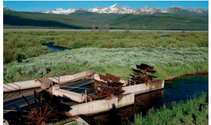
Fish screens on irrigation diversion in the upper Salmon River basin.
